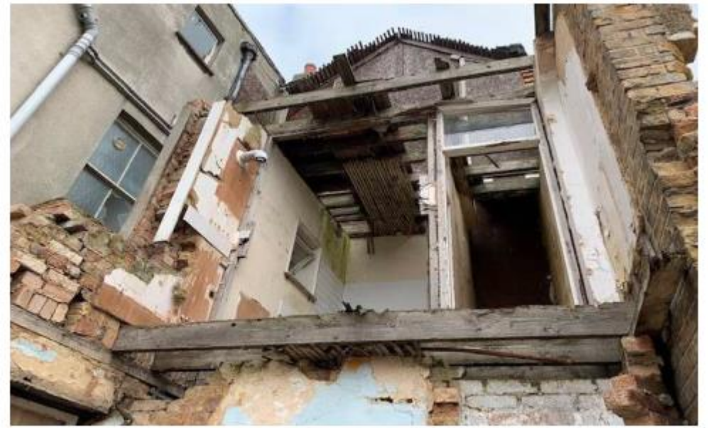
Fig 1.9.15 // Photo outside of the building, Rear elevation
