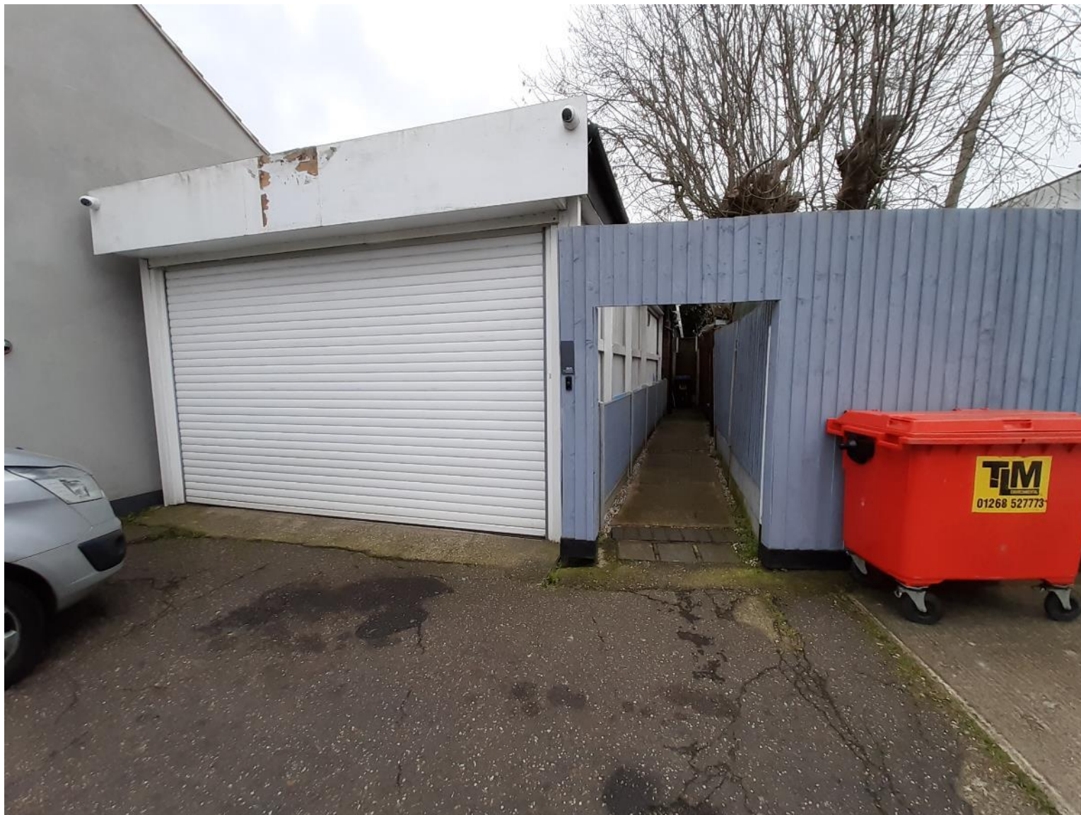
Neighbouring site – Previous entrance point for the unit
