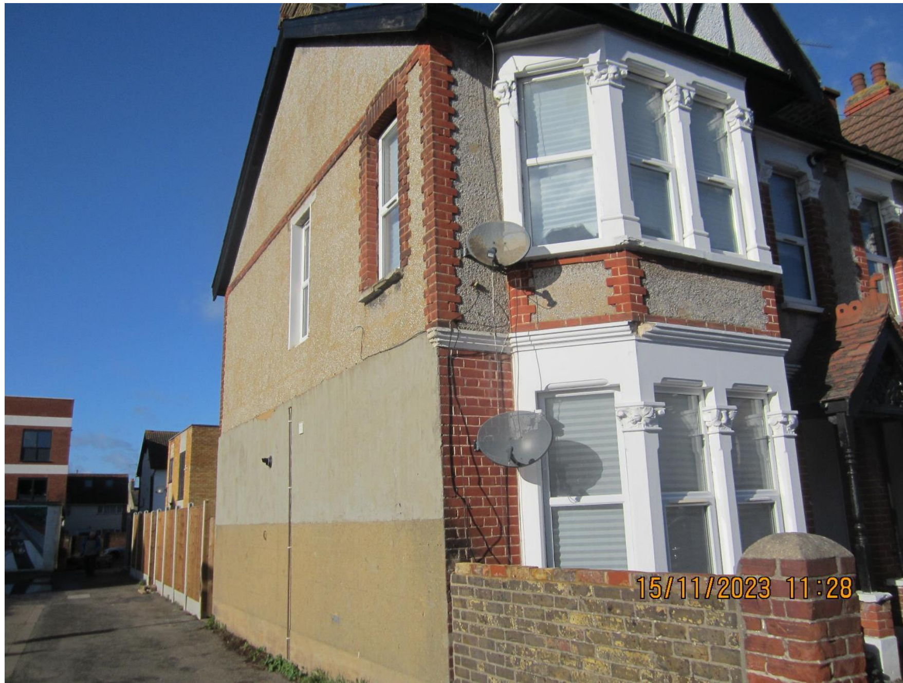
The flank elevation of the building at the site
