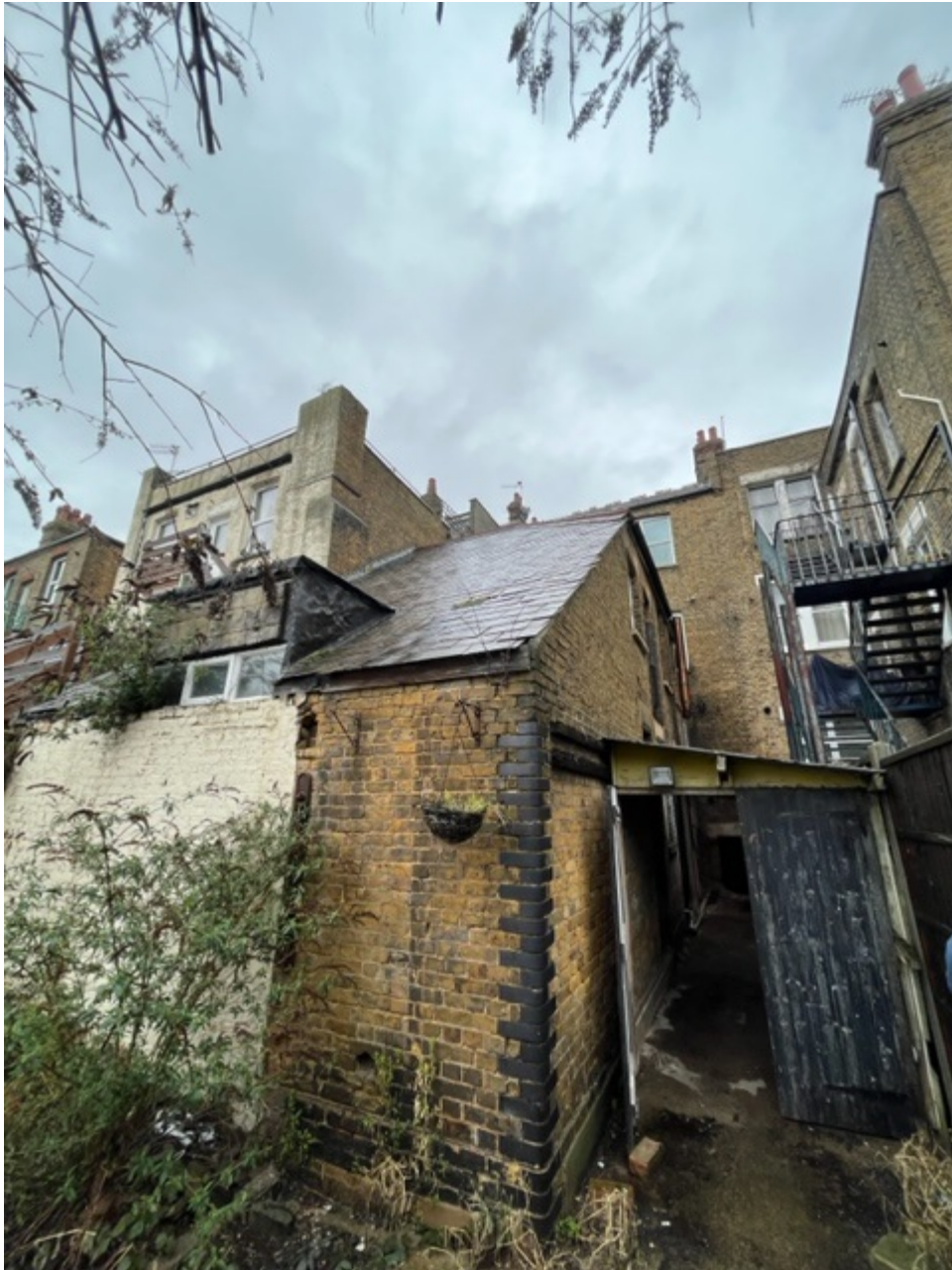
Rear of site and neighbour to east
