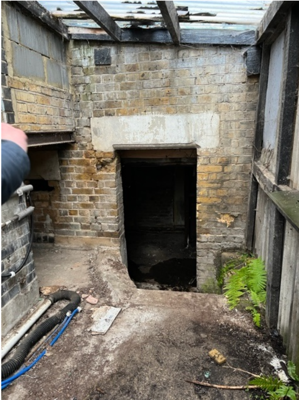
Access to existing basement
