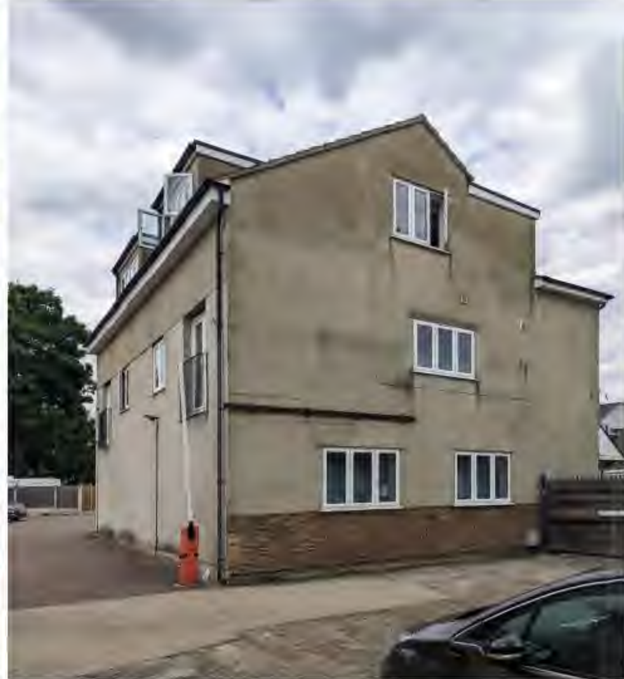
West and South Façade
