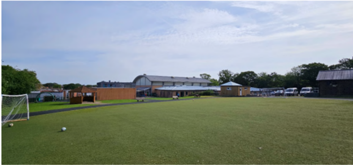
View looking back towards the main building of the school – looking North
