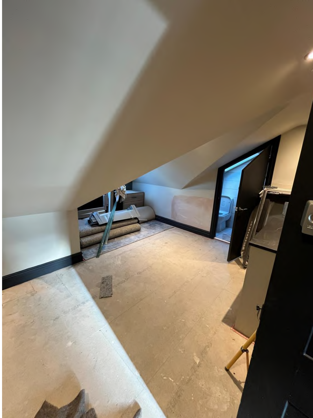
Roof room to front
