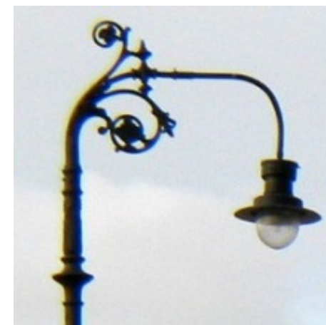
Original, decorative cast iron brackets make a positive contribution to the streetscene in the Clifftown Conservation Area
