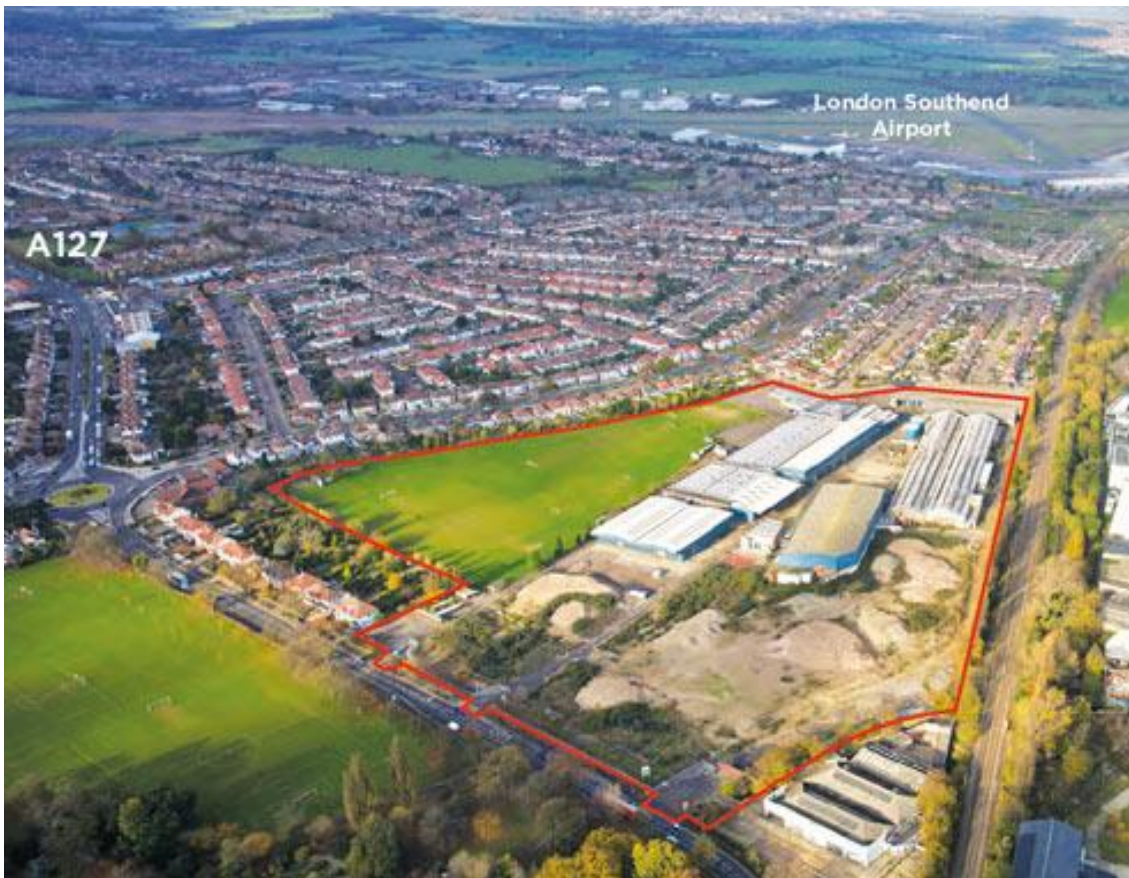
Aerial photo of site (note site now cleared)
