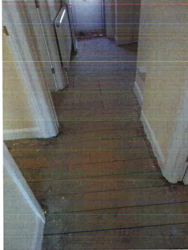
Inside the property was cleaned and restored prior to refurbishment
