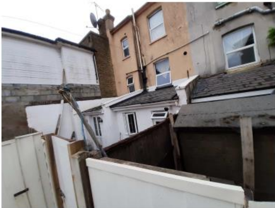
Neighbouring properties to the north-west
