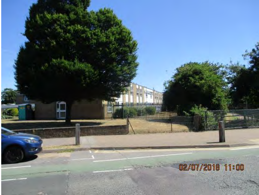
FRONT HOUSE SOUTH / EAST WITH PRITTLE BROOK ON RIGHT
