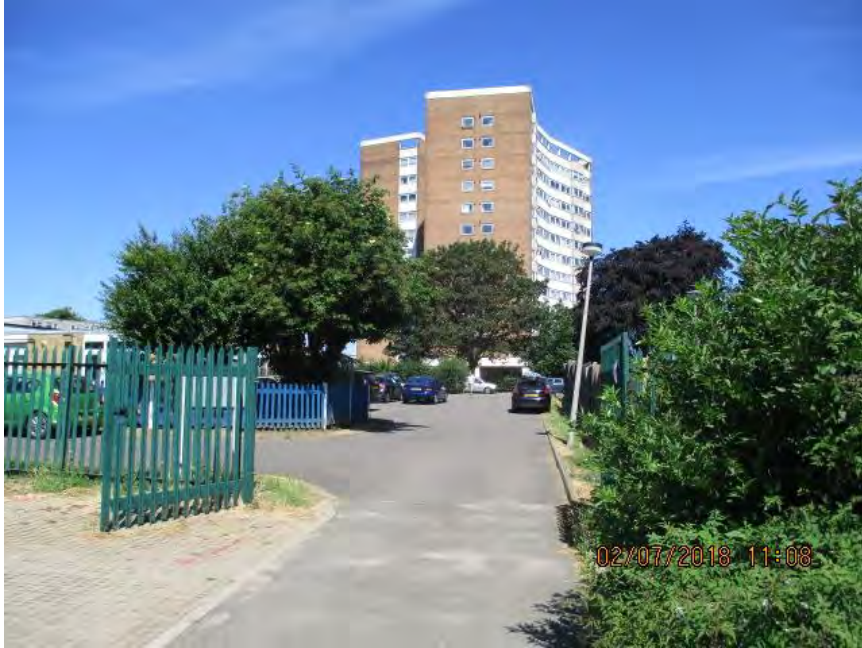
FROM REAR OF PRIORY HOUSE TO BURR HILL CHASE
