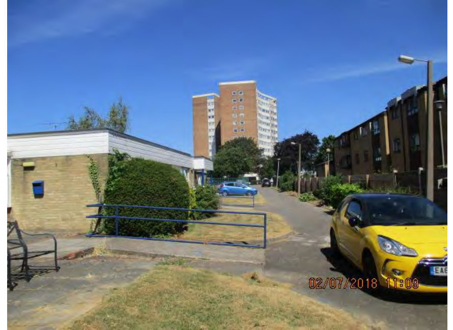
FROM REAR OF PRIORY HOUSE TO BURR HILL CHASE WITH REAR OF STEPHEN MCADDEN HOUSE TO RIGHT AND CECIL COURT CENTRE
