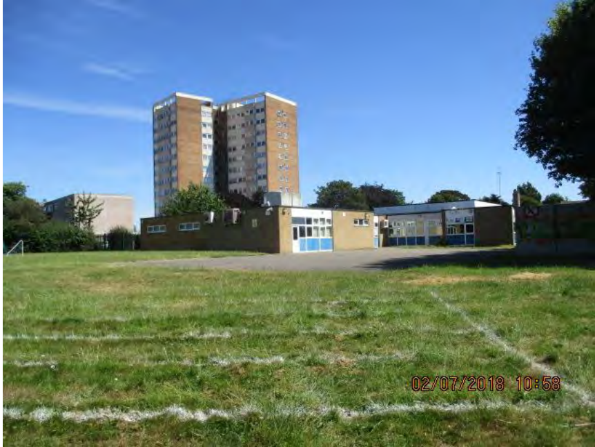
EXISTING SCHOOL BUILDING
