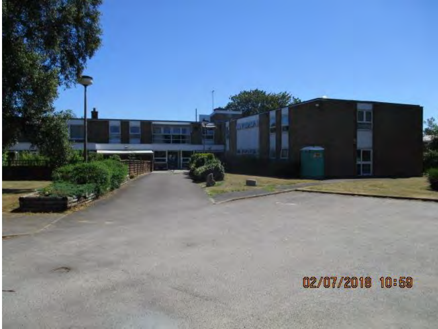
PRIORY HOUSE FRONTAGE (SOUTH ELEVATION)
