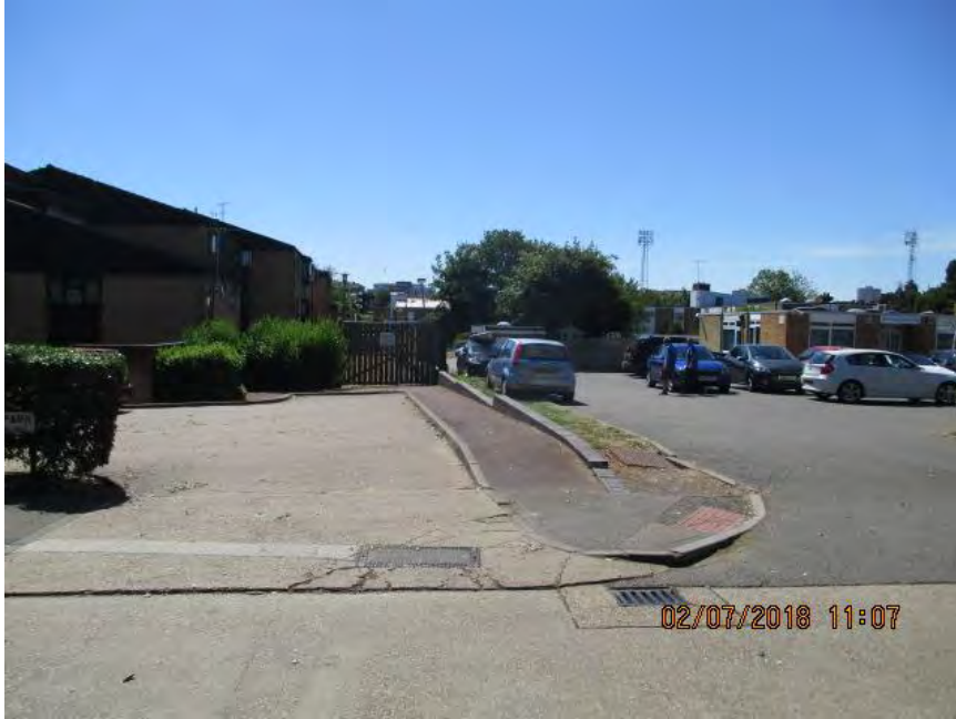
FROM BURR HILL CHASE LOOKING SOUTH WITH PRIORY SCHOOL ON RIGHT AND STEPHEN MCADDEN HOUSE ON LEFT
