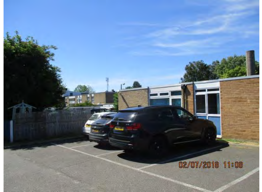
PRIORY SCHOOL EAST
