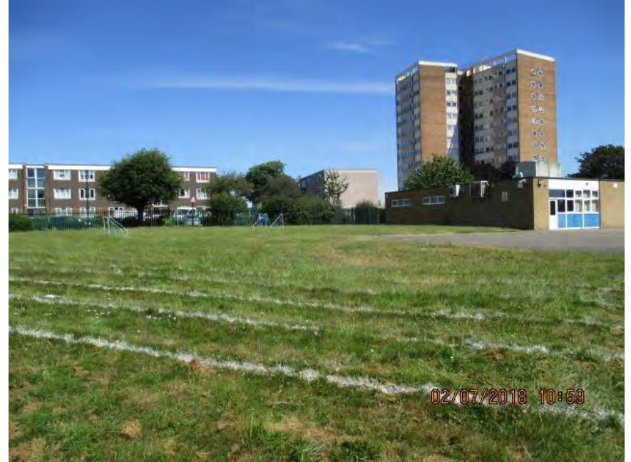
EXISTING SCHOOL BUILDING WITH BURR HILL CHASE PROPERTIES TO LEFT AND CECIL COURT TOWER ON RIGHT
