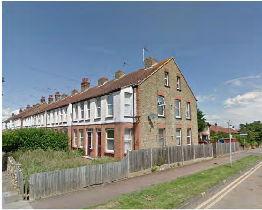
LOCATION A WITHOUT POLE
