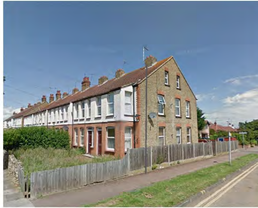
LOCATION A WITH POLE
