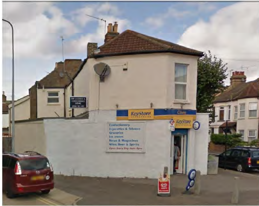
LOCATION A WITHOUT POLE
