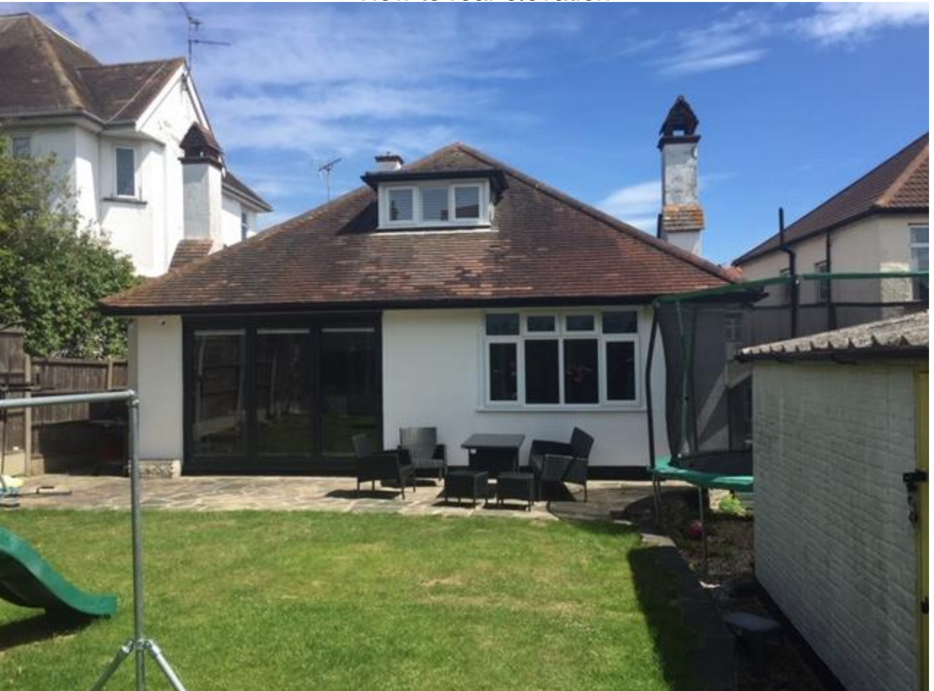
View to rear elevation
