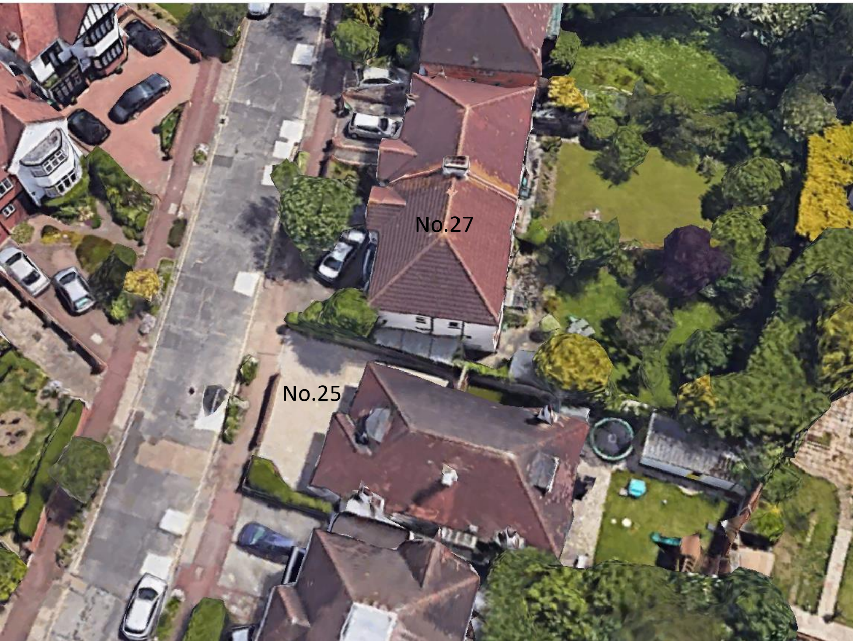
View to position of No.25 slightly behind No.27 (to the south)
