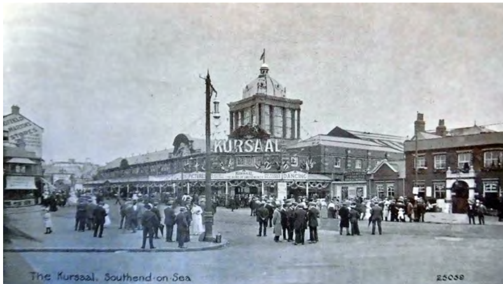
Postcard of the Kursaal, 1910. The Minerva public house features an elaborate stuccoed door case. This photograph is from before the ball finials were added to the parapet or the front elevation rendered. The single-storey building to the north has been added. (Reproduced courtesy of the Essex Record Office: D/DS 206/358)
