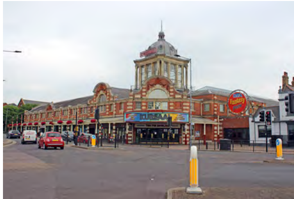
The front elevation of the Kursaal, comprising the corner range and the long east range, and the south range
