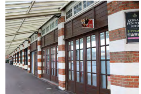
Modern windows inserted into the arcade on the west elevation
