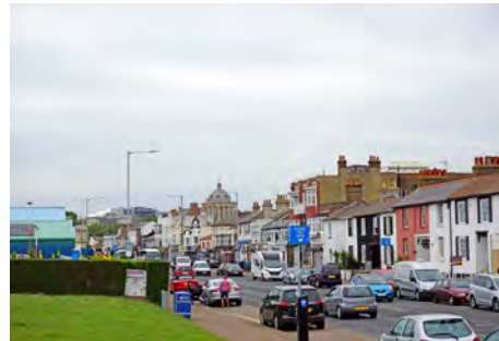
View of the cupola of the Kursaal from further east on Eastern Esplanade
