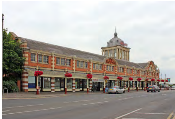
The west range of the front elevation
