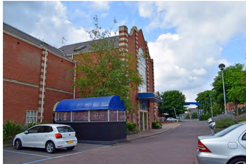
North elevation with entrance to Casino and smoking shelter
