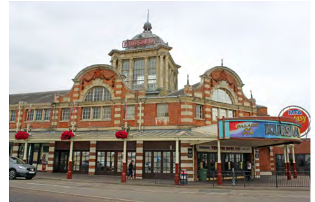
The corner range of the front elevation
