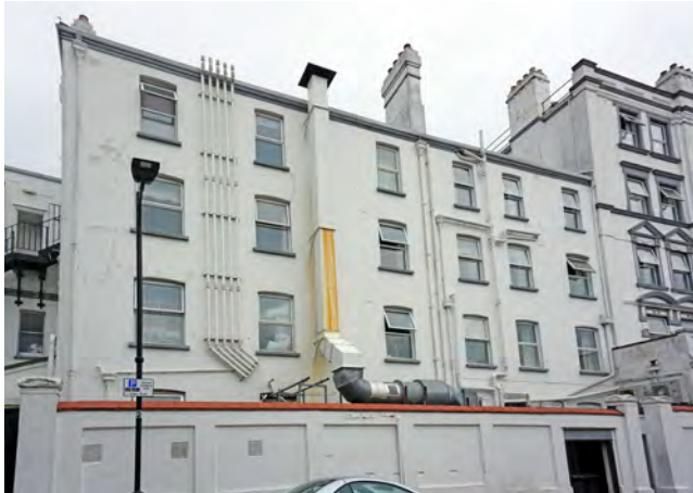
Intrusive ducting and pipework on the side of the Westcliff Hotel (2019)
