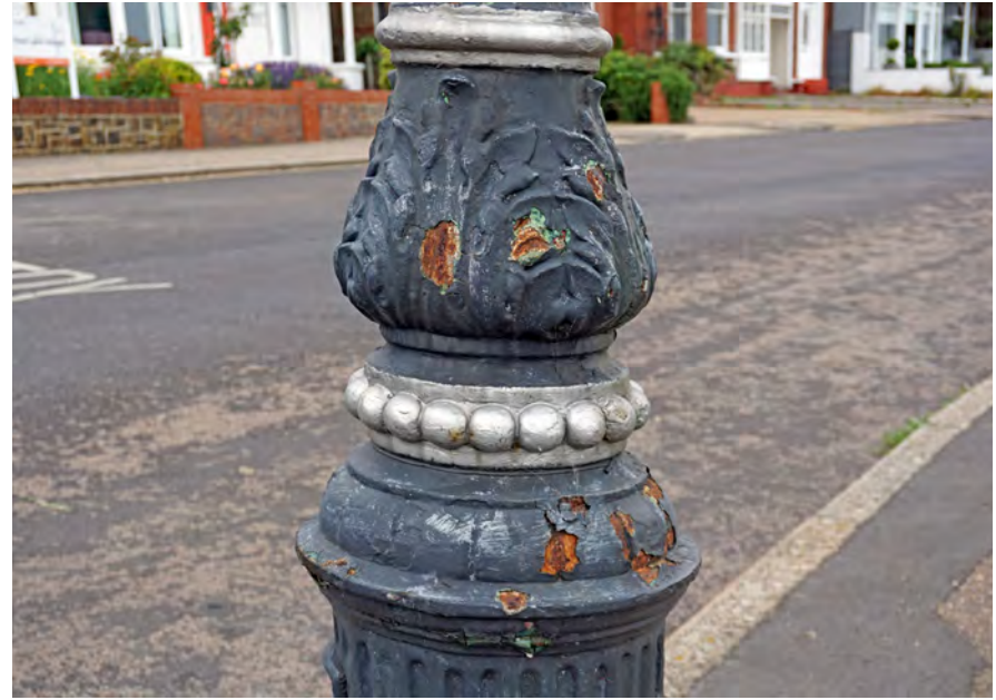
Deterioration of paintwork on historic lampposts (2019)
