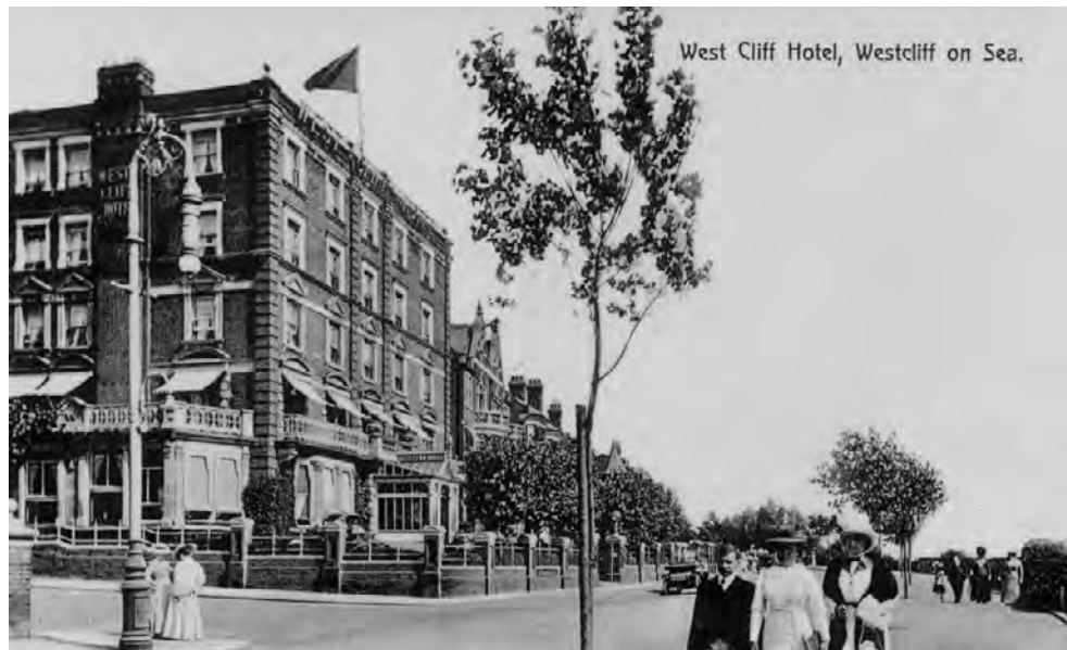
Early-20th century photograph of the Westcliff Hotel after the addition of a glazed entrance porch and side bay window extension but before the brickwork was rendered
