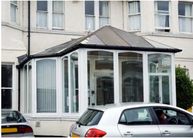
Inappropriate porch on Westcliff Avenue (2019)
