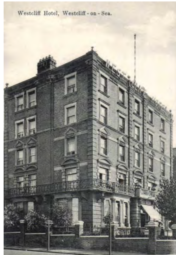
Late-19th century photograph of the Westcliff Hotel, showing the building before the entrance porch and side bay window extension were added and before the brickwork was rendered
