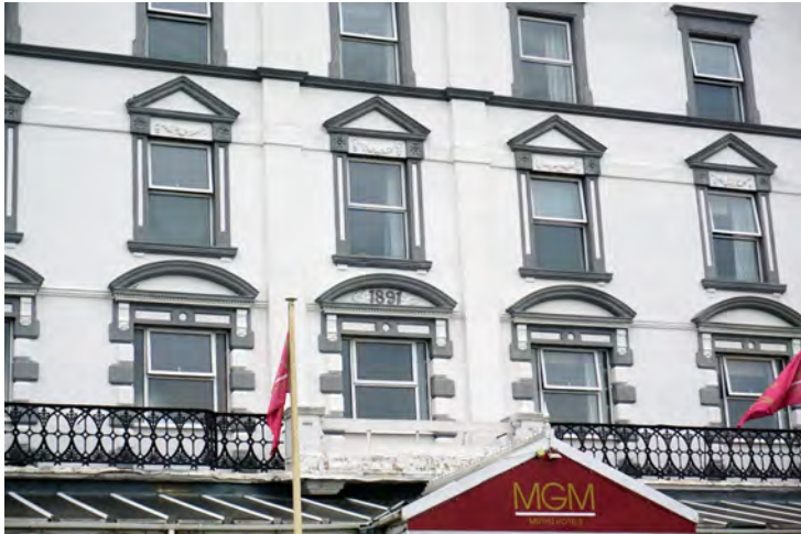
uPVC windows and painted brickwork on the Westcliff Hotel (2019)
