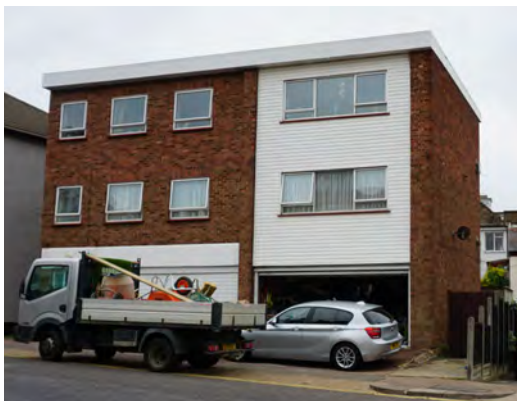
2a and 2b Westcliff Avenue which are not an appropriate design for the character of the Conservation Area
