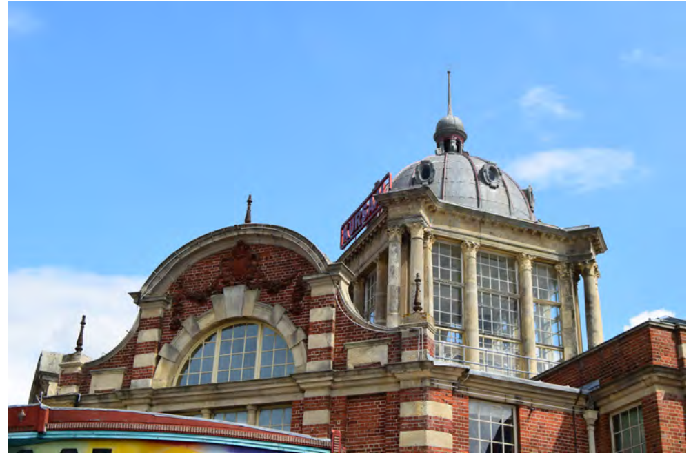
The square-based tower and dome
