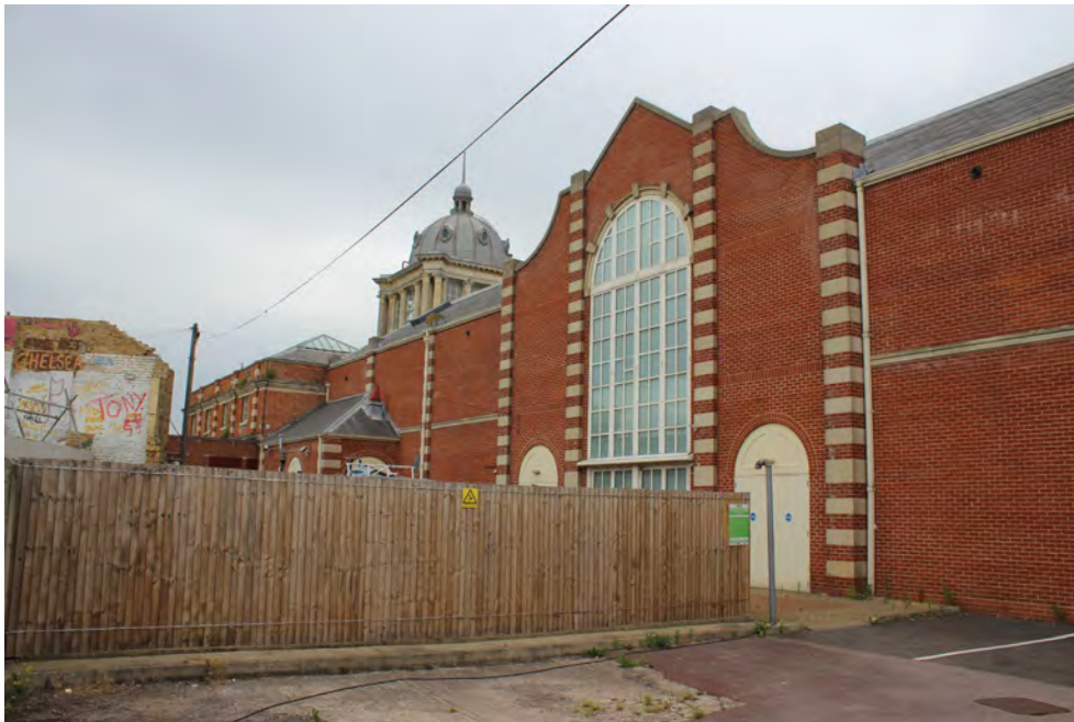
The south range comprising the historic bar range on the left and the re-fronted theatre range on the right
