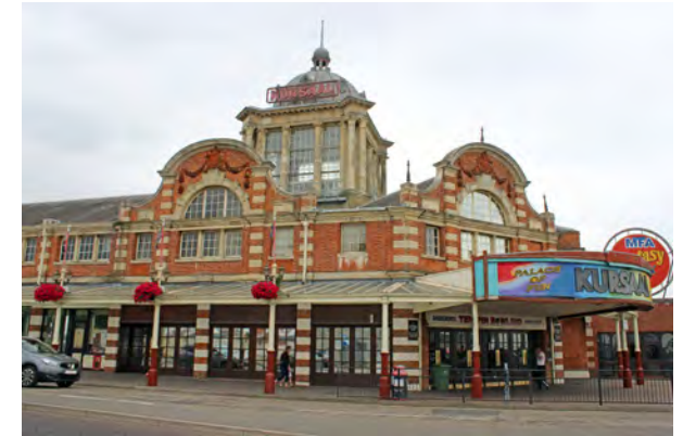
The corner range of the front elevation
