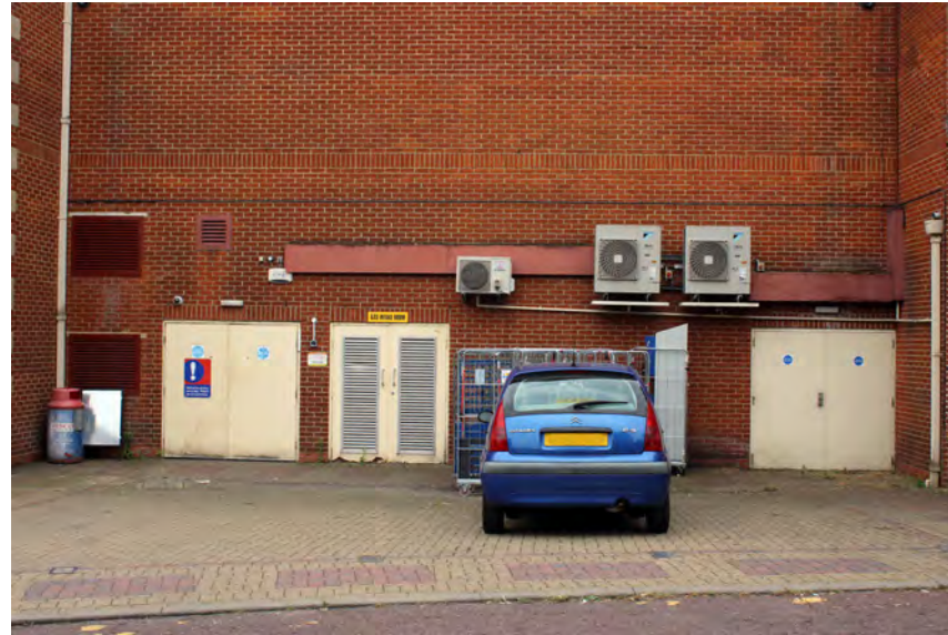
Ventilation grilles and exhaust flues in the north elevation
