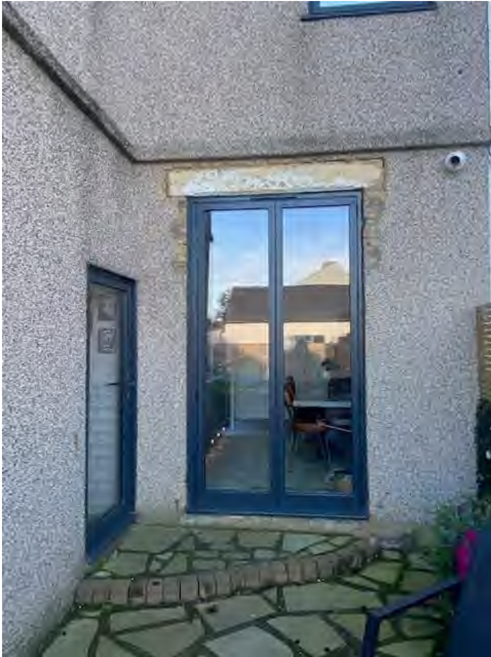
REAR WINDOWS OF 143 (KITCHEN/DINER AND UTILITY ROOM ON FLANK)
