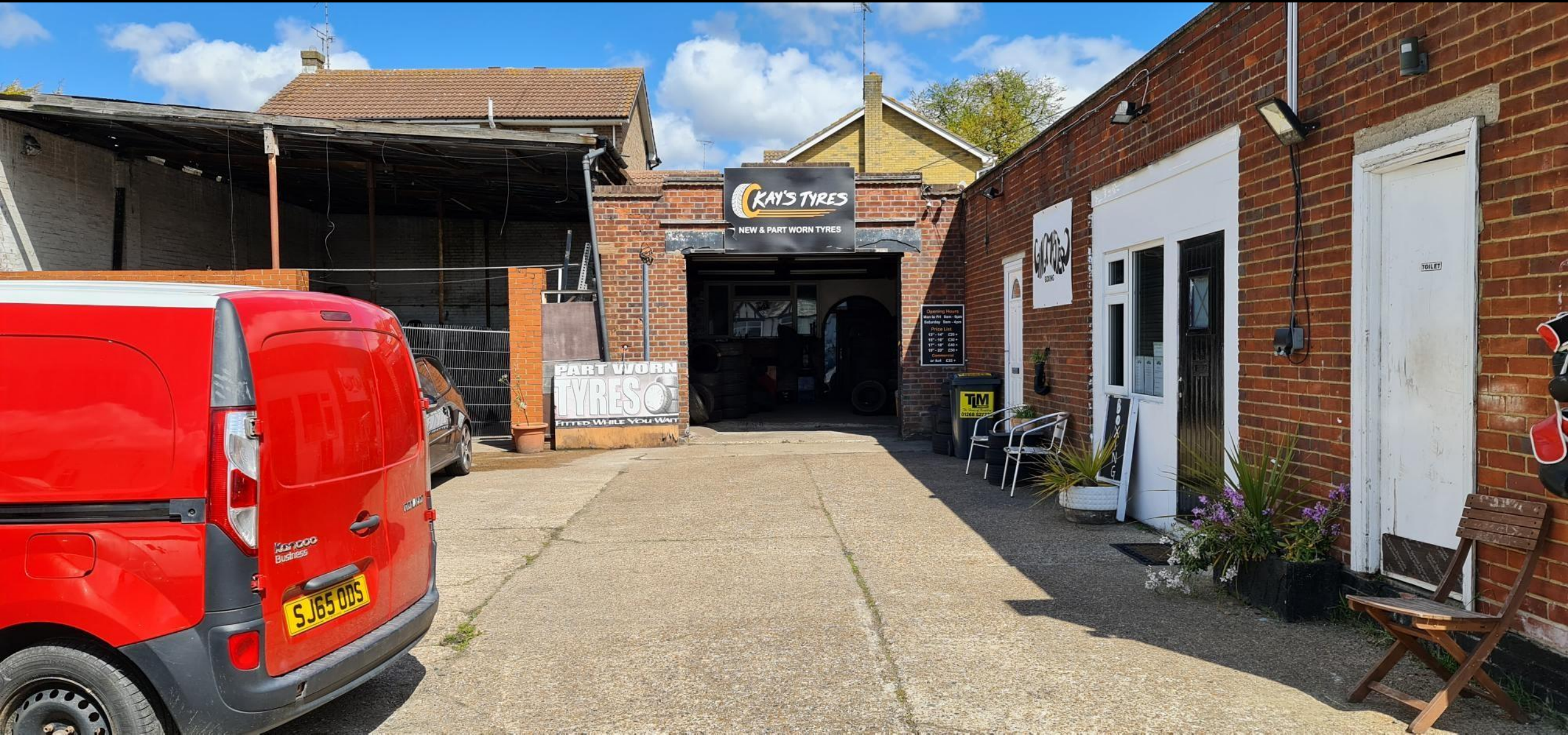
Nos.22-24 The Rodings to rear of site, with gym at right, prior to external alterations
