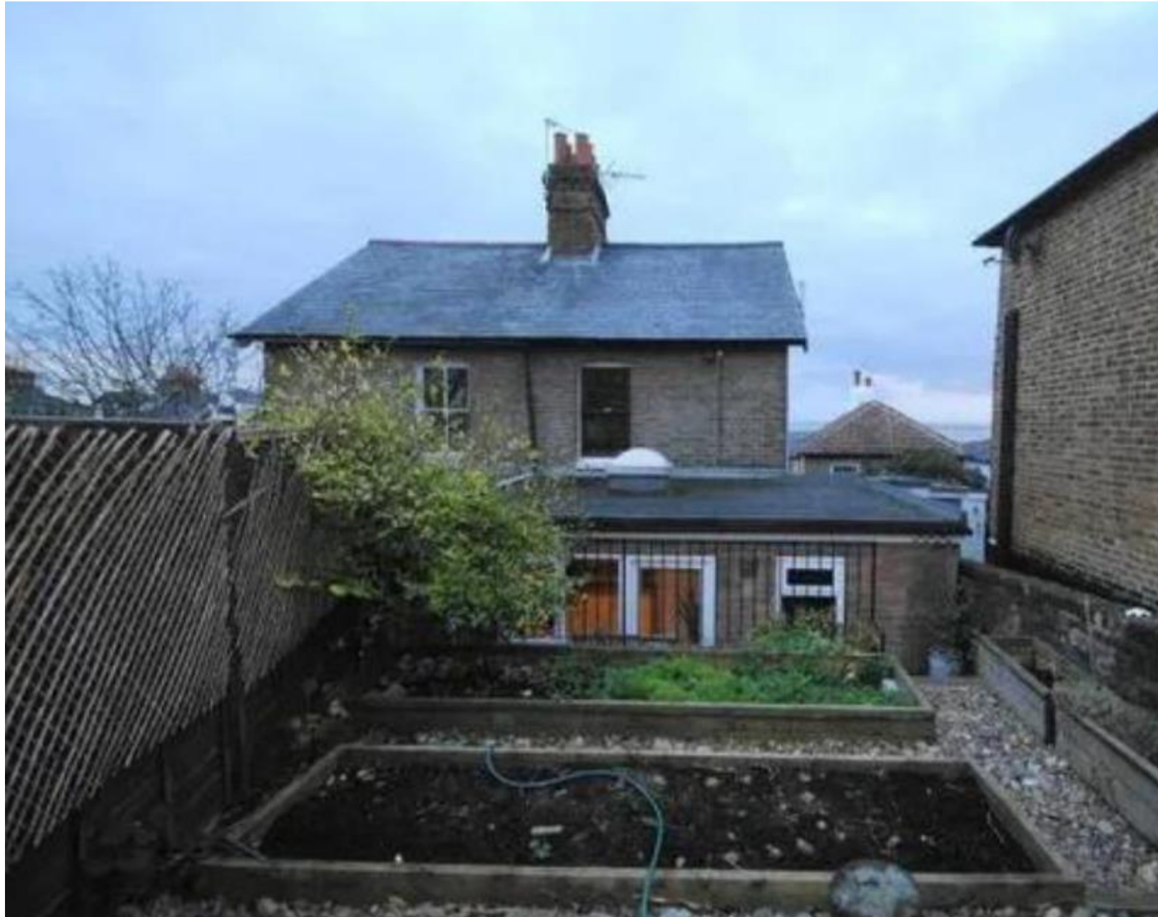
Rear elevation before
