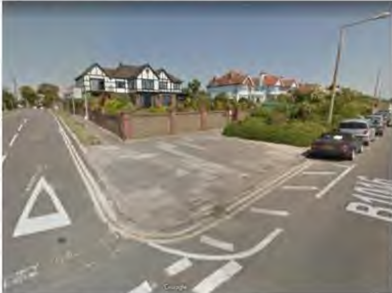
View from South West corner
