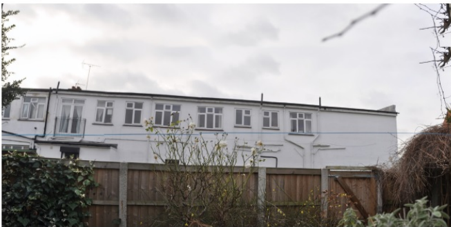
Existing View from 10 Grasmear Avenue
