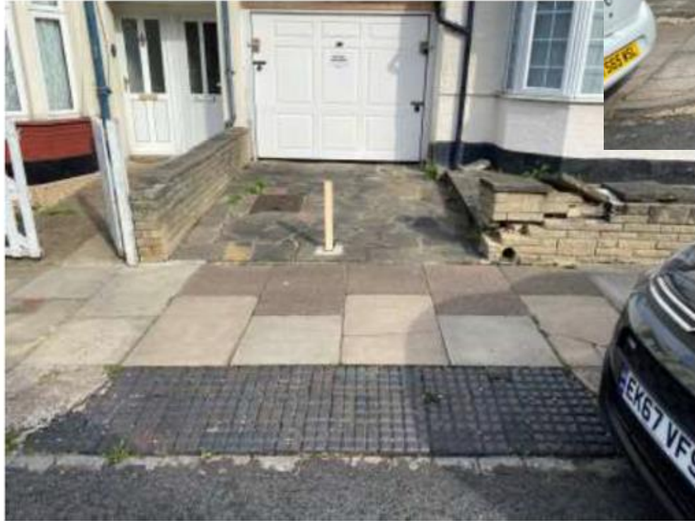
Existing crossover to garage
