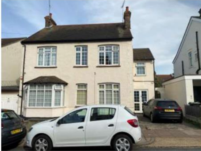
Application Site Front
