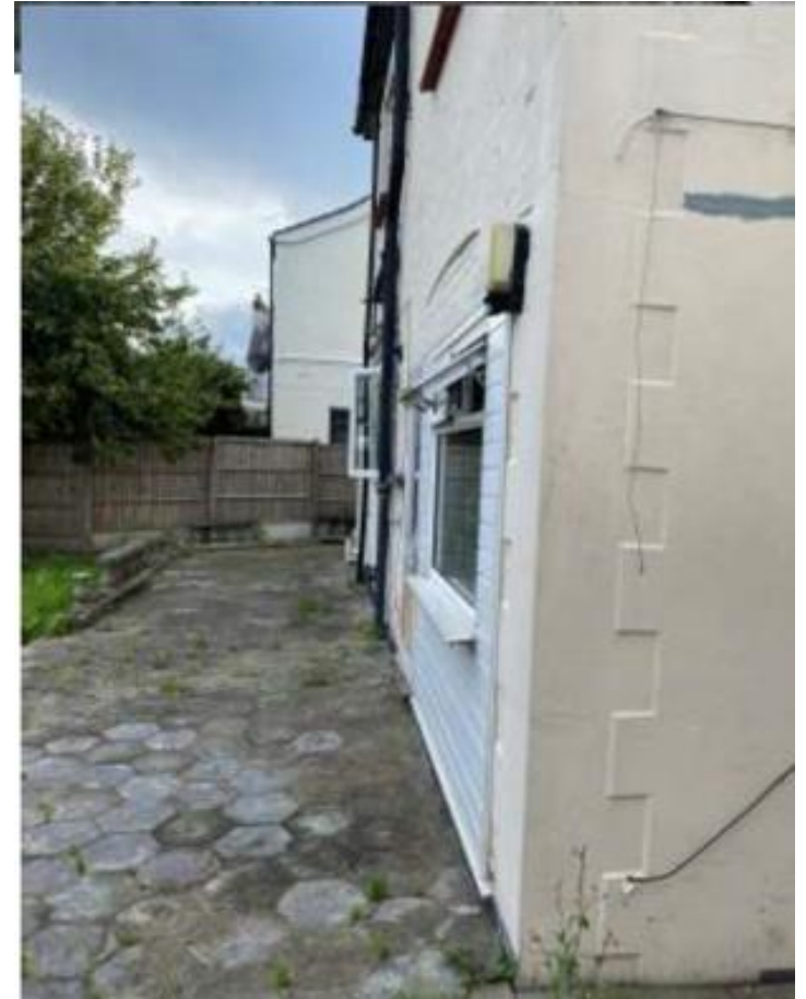
Rear Looking South
