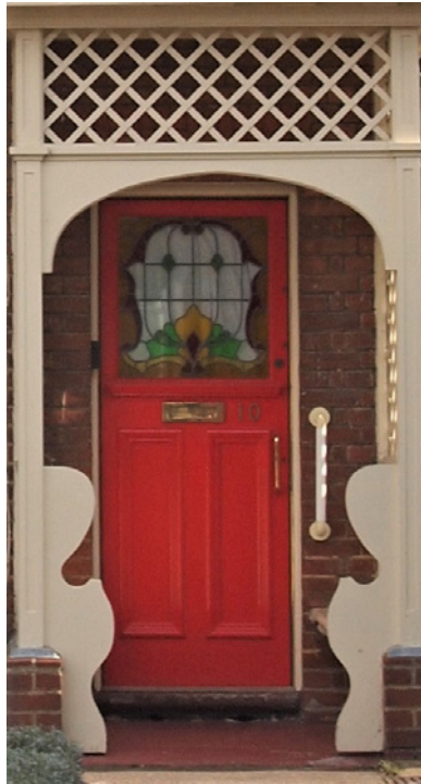
Door and entrance porch to No.10
