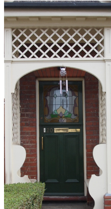
Door and entrance porch to No.20
