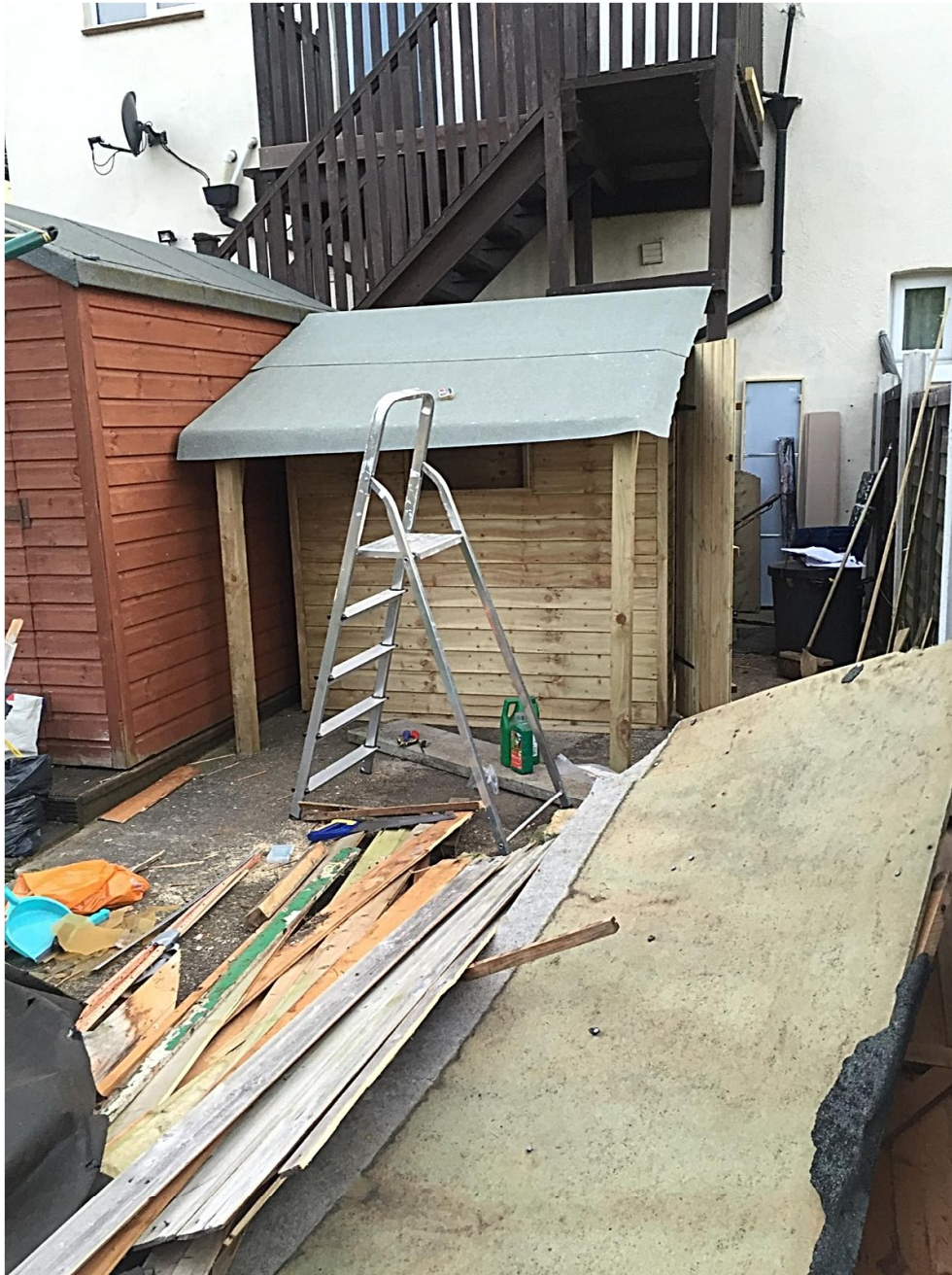
Existing - Before construction after old shed was removed
